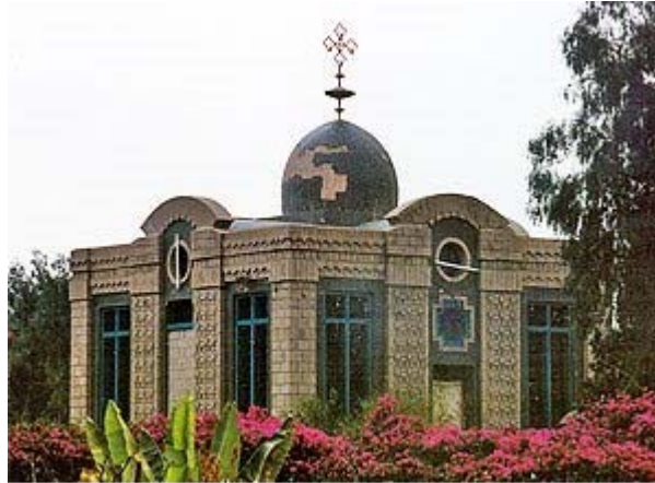
Saint Mary of Zion Church in Axum, Ethiopia where the Ark of the Covenant is supposedly housed.
